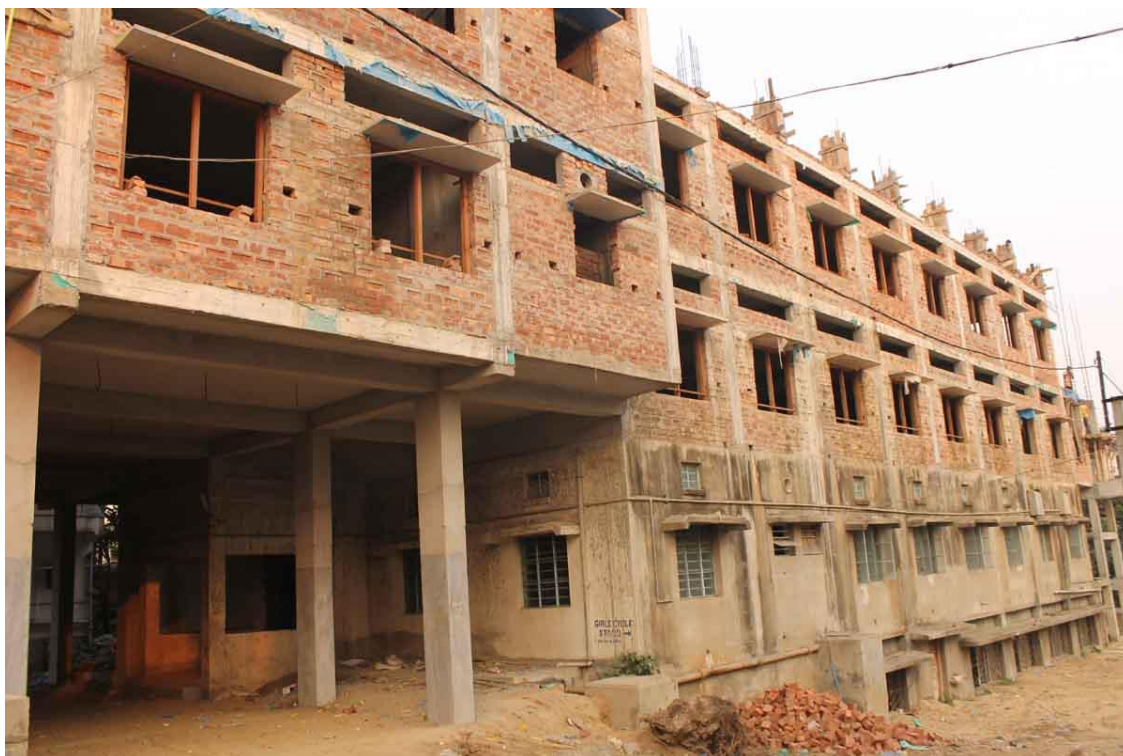
New expansions of the already existing PG Building
